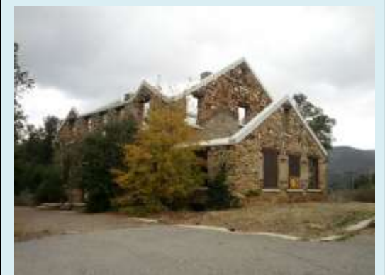
Support our campaign to rebuild The Dyar House which will house our Sector Headquarters, Visitor Center, Museum, Gift Store, and Volunteer Ready Room. Photo by Michele Hernandez
